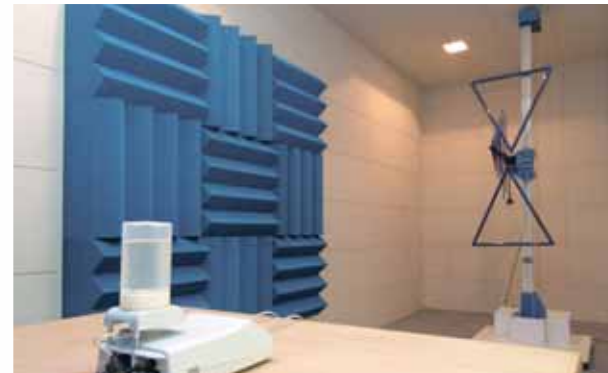
Developing safe products that comply with European EMC standards with an anechoic chamber installed to measure electromagnetic waves.
